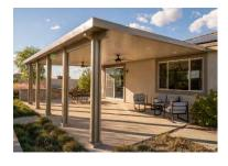
2.9 Balcony Cover: A single story architectural projection located at balcony levels that provides partial weather protection but remains open on three sides. One end of the cover is supported by the building while the opposite end is supported by a post and beam configuration.
