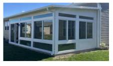
The enclosure is both attached to the building and self-supported.
